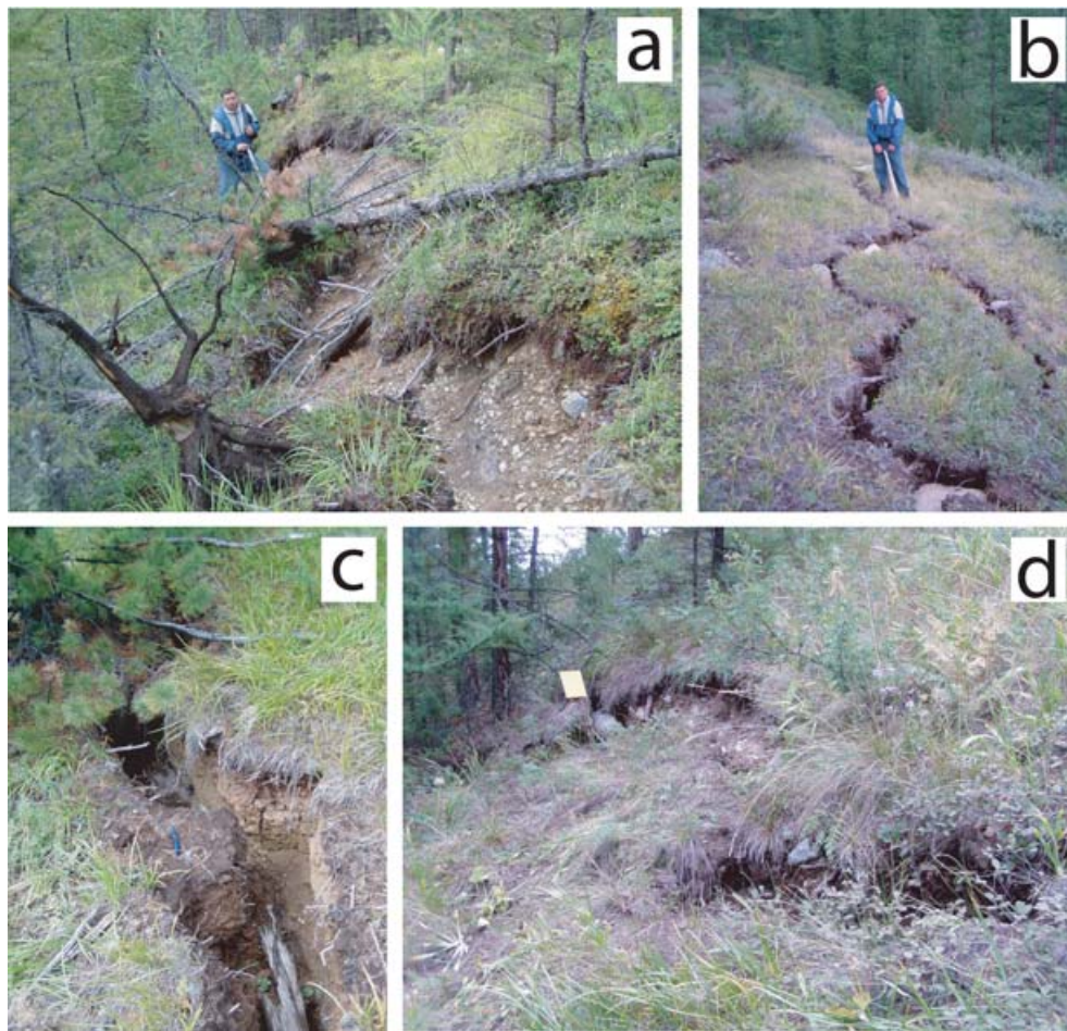
Figure 3. Field photos of earthquake ruptures in the southern Kurai depression, denoted by a star in Figs 2, 6 and 8. (a) 50^{\circ} 08.273'N 87^{\circ} 48.577'E , facing 030^{\circ} . The fissure strikes 030^{\circ} and is offset vertically by 40 cm, up to the SE. (b) 50^{\circ} 08.342'N 87^{\circ} 48.582'E , facing 180^{\circ} . These fissures strike N–S along a small ridge. (c) Detail of a fissure on the same ridge as (b) with a pen for scale, pointing N (up). The fissure is 35 cm wide and offset vertically by 10 cm, up to the E. (d) Photo at 50^{\circ} 08.532'N 87^{\circ} 48.632'E , facing 005^{\circ} , with notebook for scale. This fissure strikes \sim NW for 30 m along the western flank of another small ridge.
